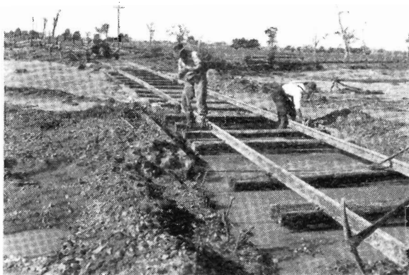
The bridge that was silted up
