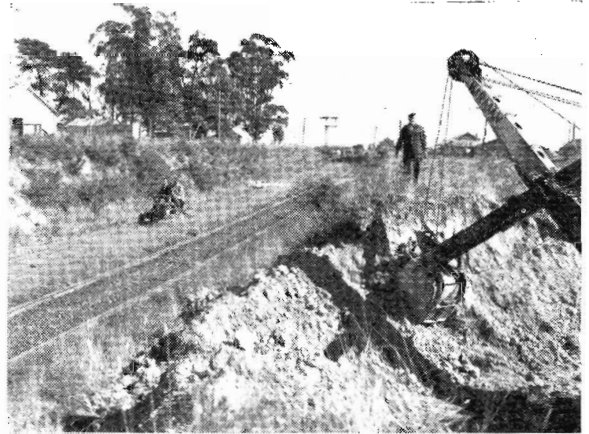
Power shovel excavating for junction with main line
