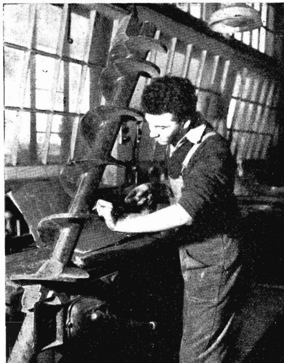
Bench work on pattern for fuel conveyor screw of Heavy Harry
