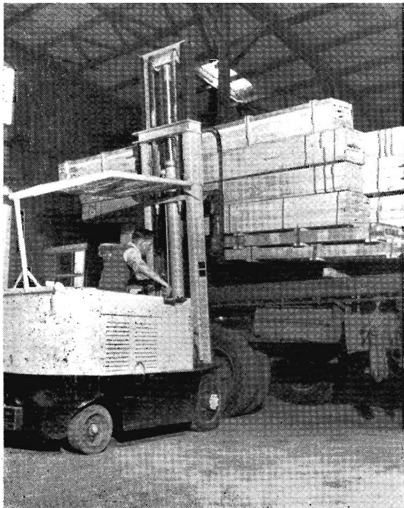
Materials are stock-piled in Brooklyn depot
