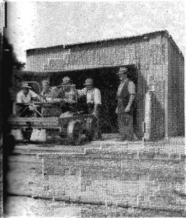
Driver A. Anderson; Labourer D. Bush; and Ganger T. O'Connor.
